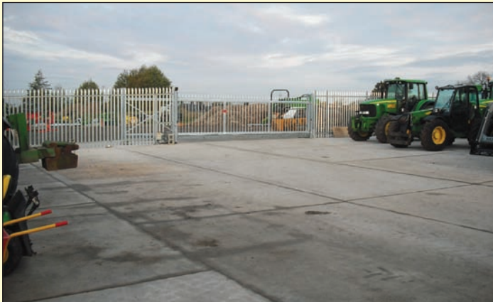
Area to the rear of the workshop, newly concreted and enclosed by security gates
