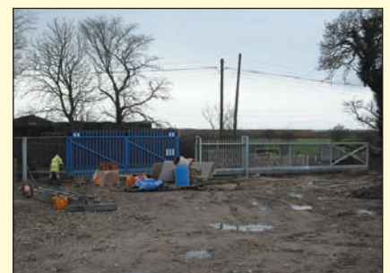
Installing the new main entrance
