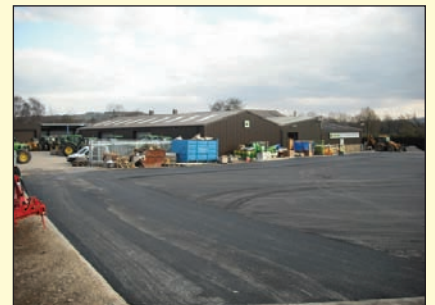
Covered in tarmac, awaiting the return of the machines
